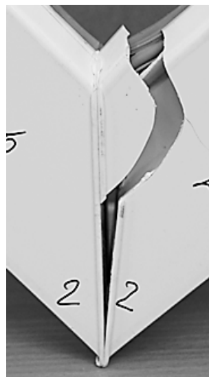
Figure 10. Corner R5 – temp. 210 °C
